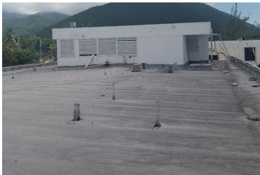
Image 9: Showing Roof for Minor Operations
