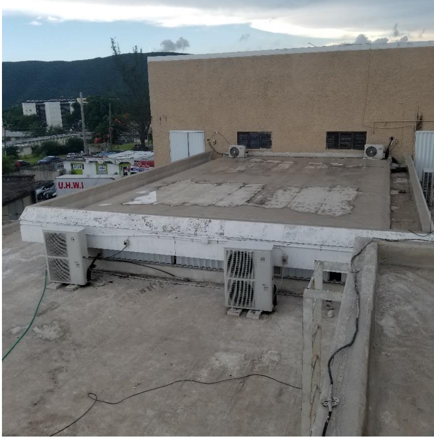
Image 40: Showing Accident and Emergency Roof
