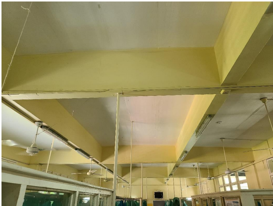
Image 67: Showing Wards 11 & 12 Soffit
