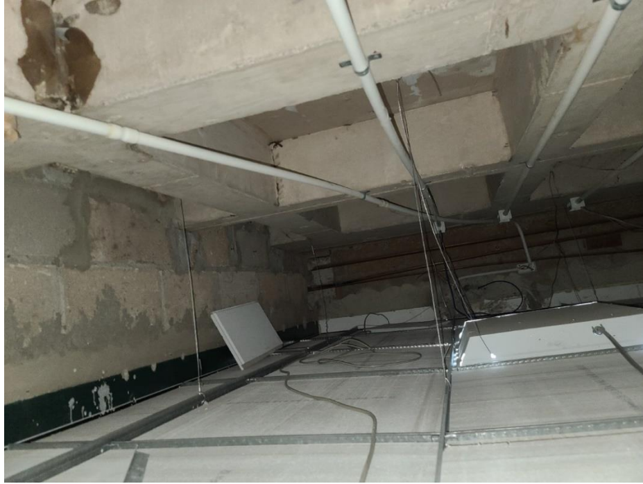
Image 24: Showing ICU A Roof Slab Soffit
