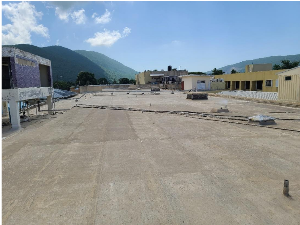
Image 25: Showing Operating Theatre 1-5 Roof
