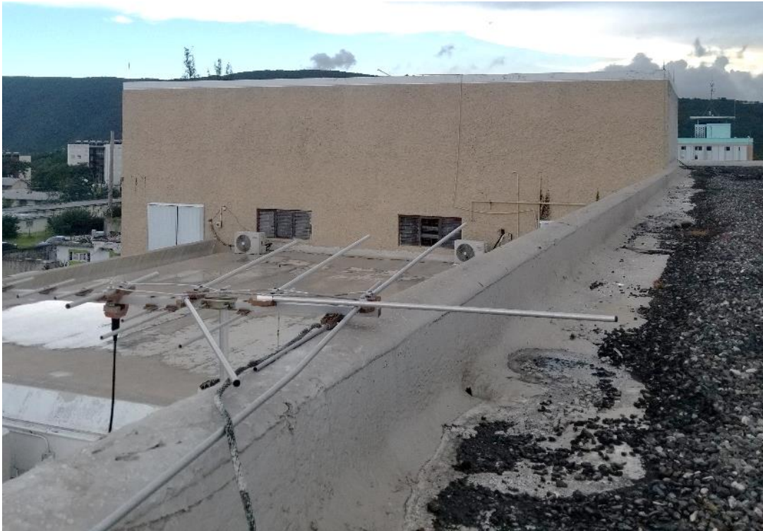
Image 39: Showing Accident and Emergency Roof
