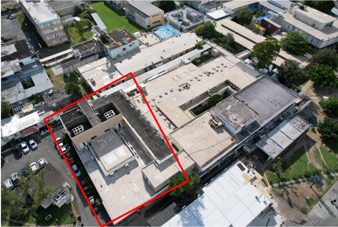
Image 42: Showing Accident and Emergency Roof
