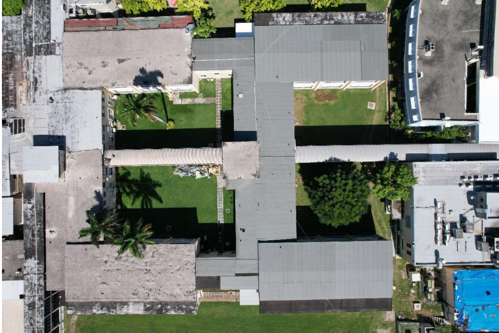
Image 60: Showing Wards 1-8 Roof
