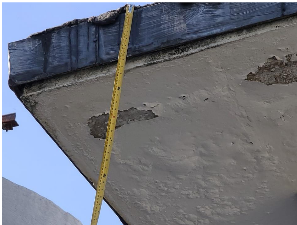
Image 75: Showing Microbiology/ Pathology Roof Slab
