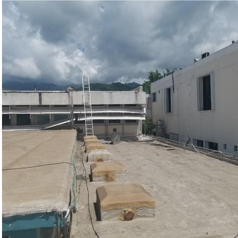
Image 48: Showing the Pharmacy Roof
