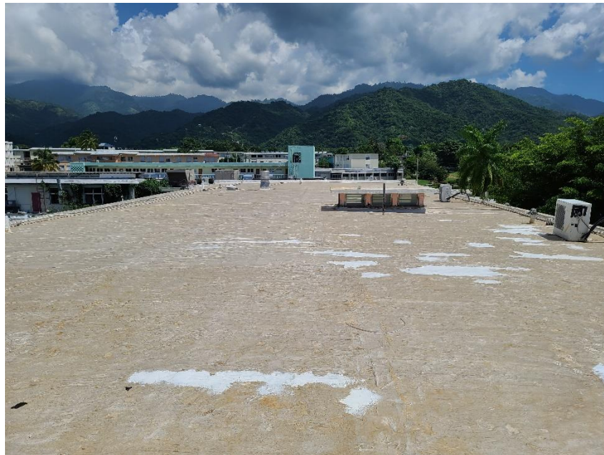
Image 71: Showing Labour Ward Roof
