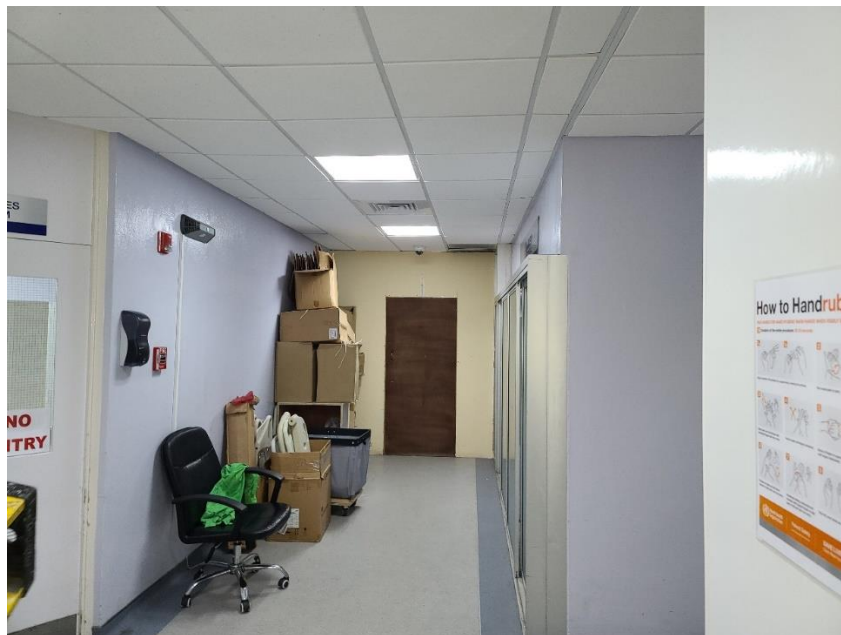
Image 41: Showing Accident and Emergency Ceiling.
