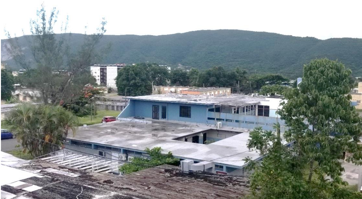
Image 38: Showing Psychiatry Ward Roof
