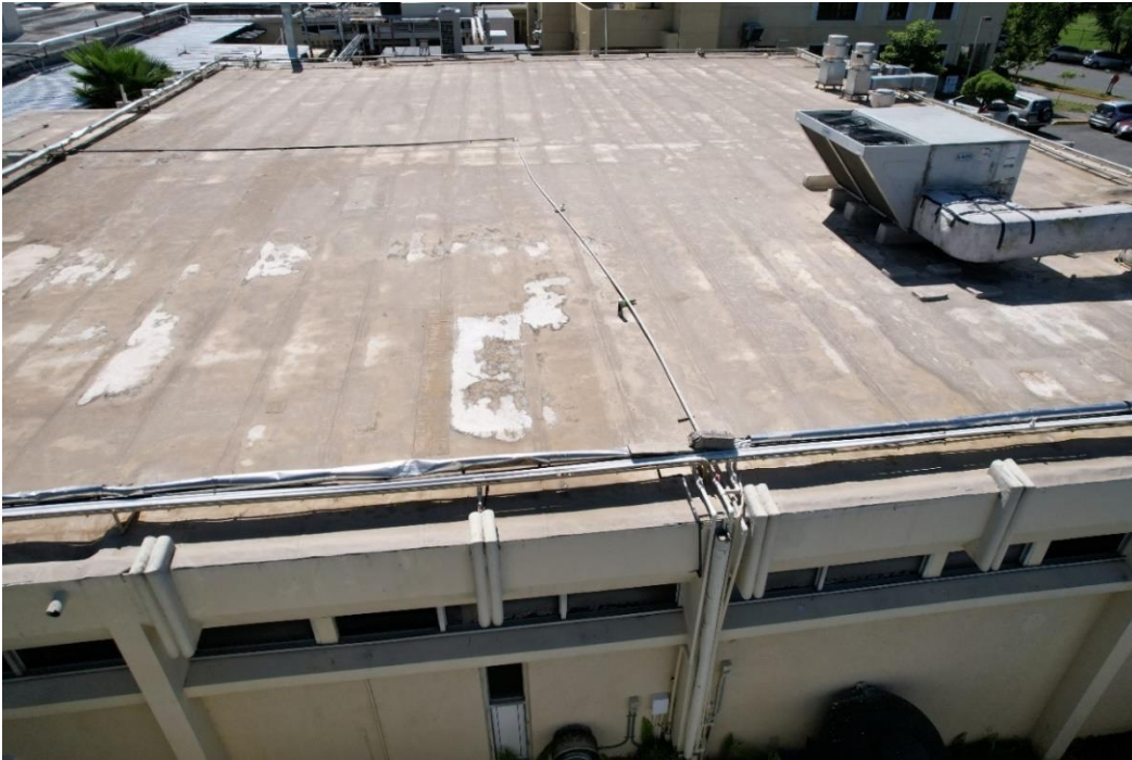
Image 22: Showing ICU A roof.
