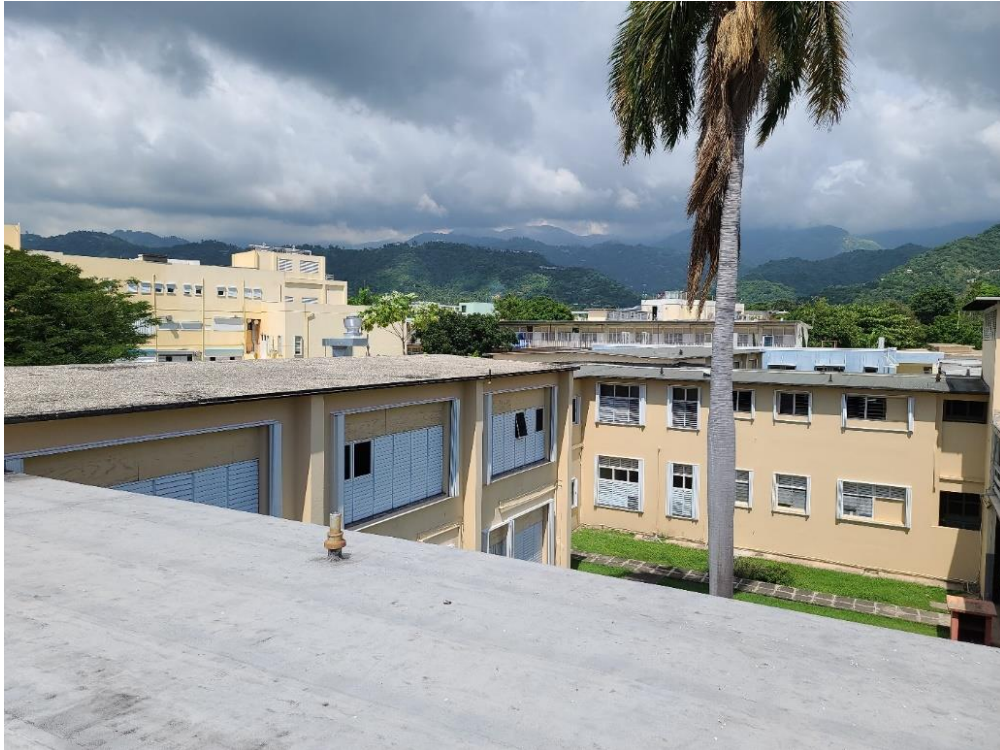
Image 58: Showing Wards 1-8 Roof
