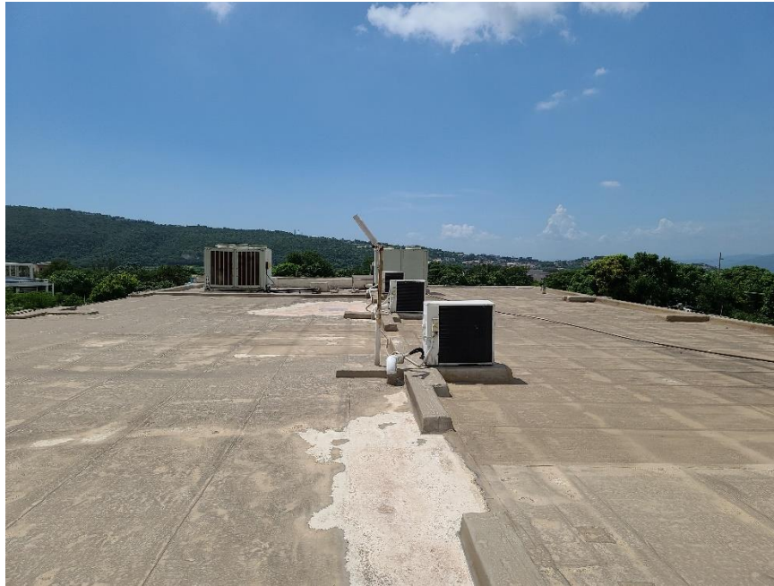
Image 80: Showing Medical Library Roof
