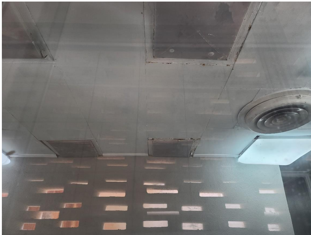
Image 29: Showing Operating Theatre 1-5 Ceiling.
