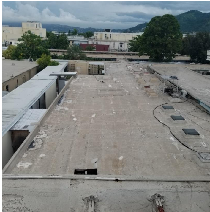
Image 46: Showing the Pharmacy roof
