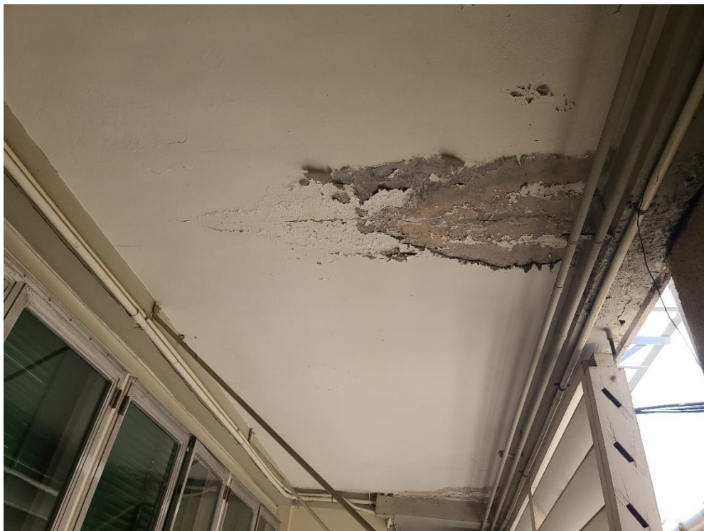
Image 26: Showing Operating Theatre 1-5 Walkway Soffit
