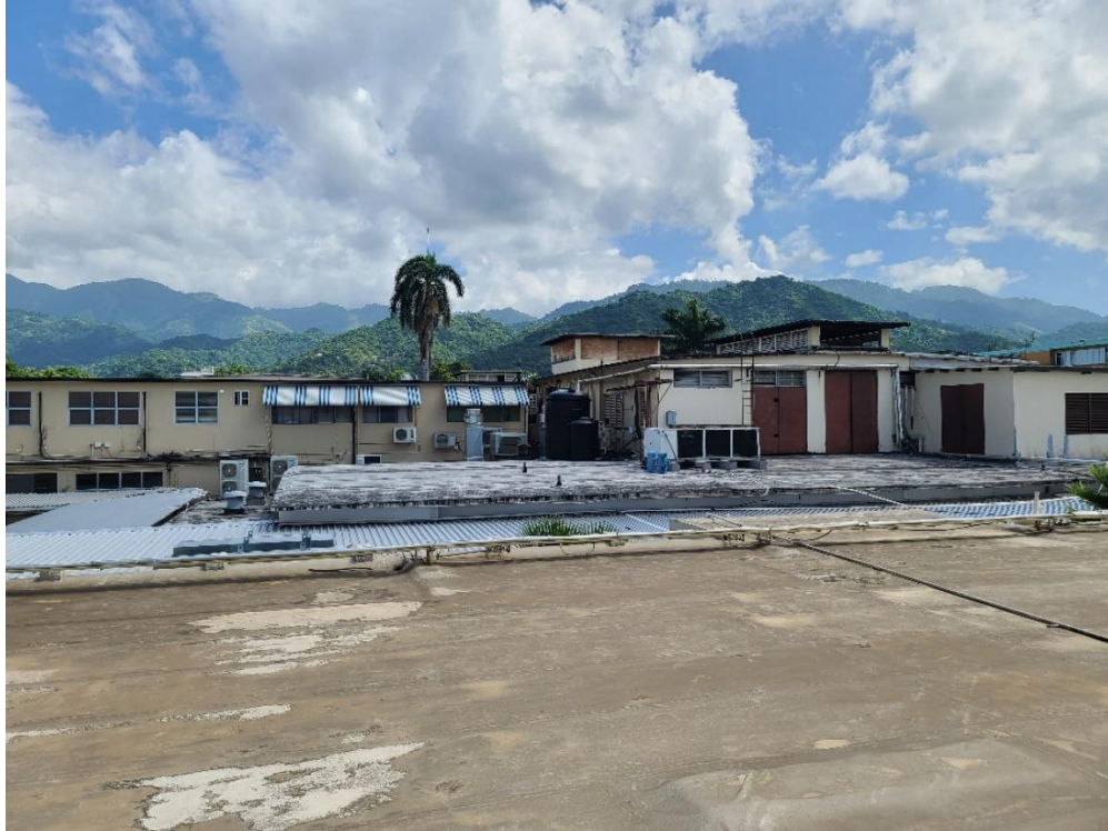
Image 28: Showing Operating Theatre Roof
