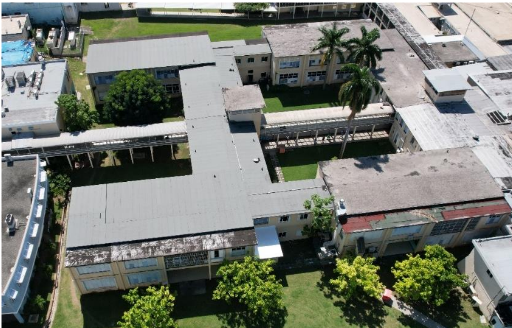
Image 59: Showing Wards 1-8 Roof
