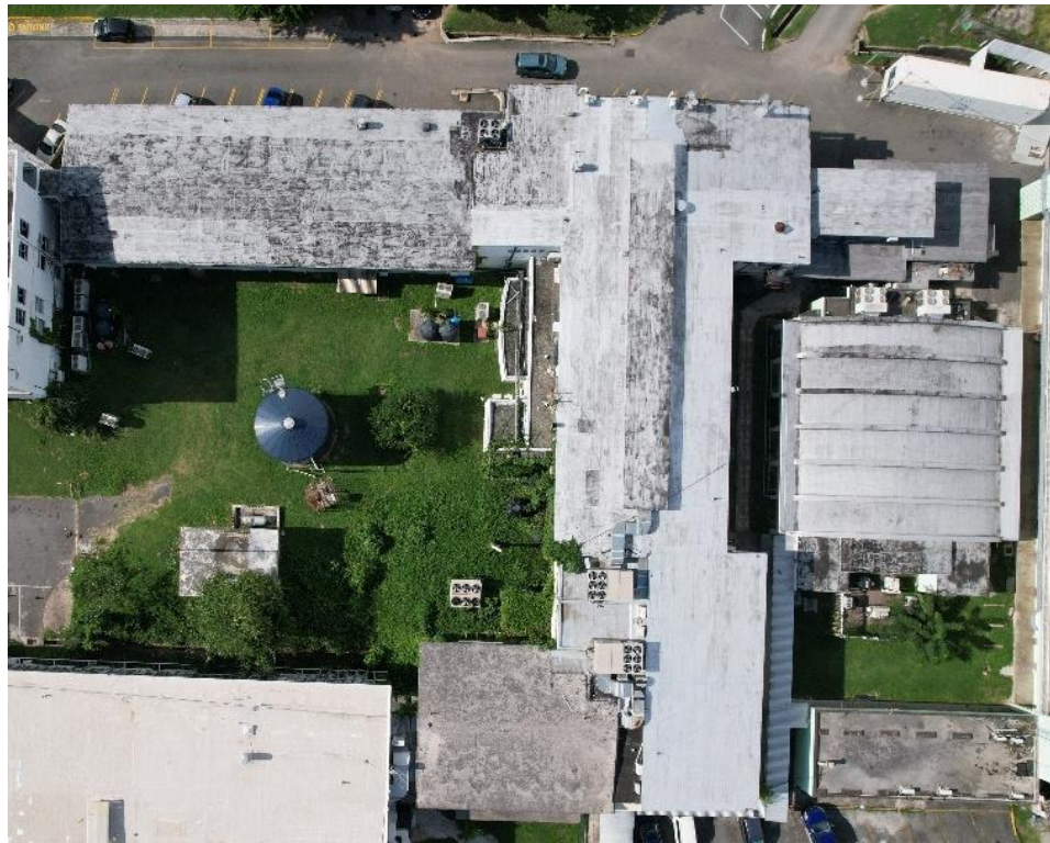
Image 77 Showing Microbiology/ Pathology Roof
