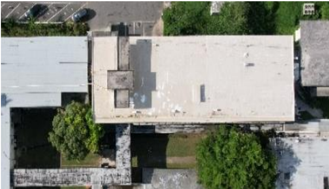
Image 73: Showing Labour Ward Roof.
