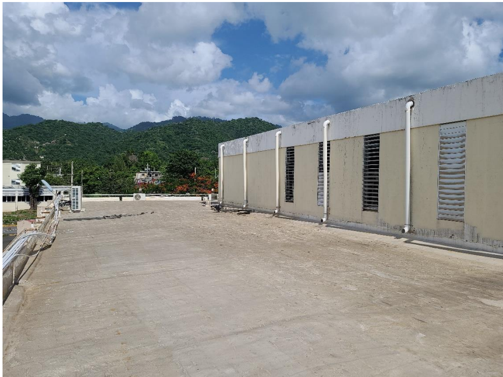
Image 61: Showing Administration Building Roof
