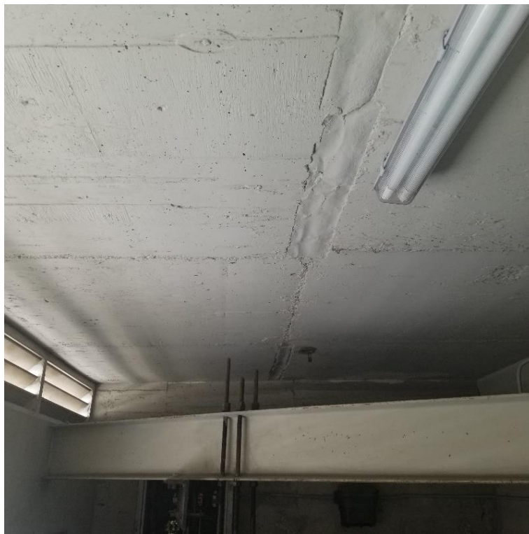
Image 45: Showing Minor Operations Soffit.
