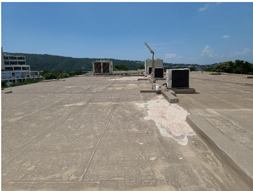
Image 81: Showing Medical Library Roof
