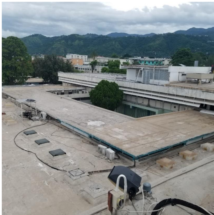
Image 47: Showing the Pharmacy Roof
