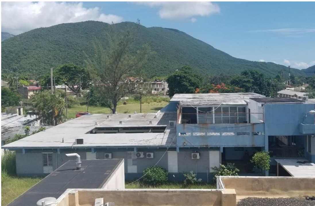
Image 37: Showing Psychiatry Ward Roof
