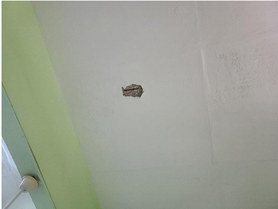
Image 66: Showing Wards 11 & 12 Soffit
