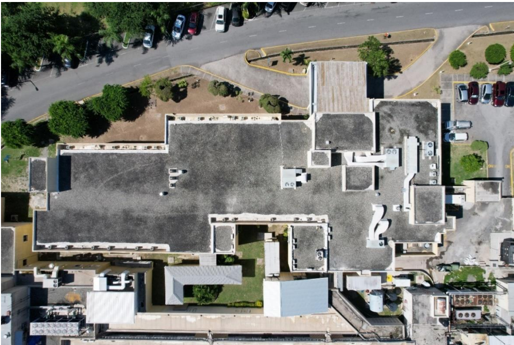
Image 21: Tony Thwaites Private Wing Building Roof.
